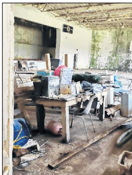
Mold on and in the Walls
