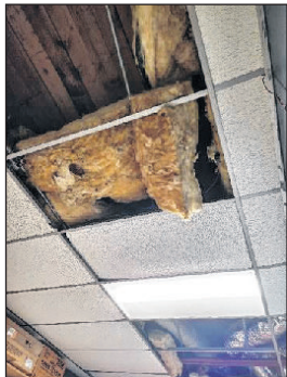
Exposed Insulation
