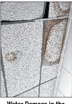
Water Damage in the Ceiling/Black Mold
